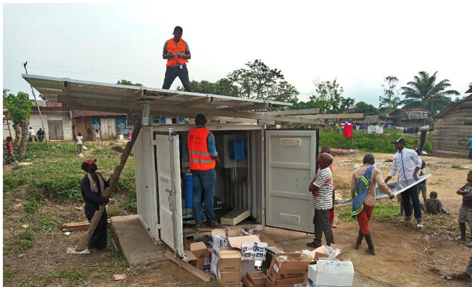
Technicians work to install an off-grid box system in Mubi as part of the Congo Power program.
